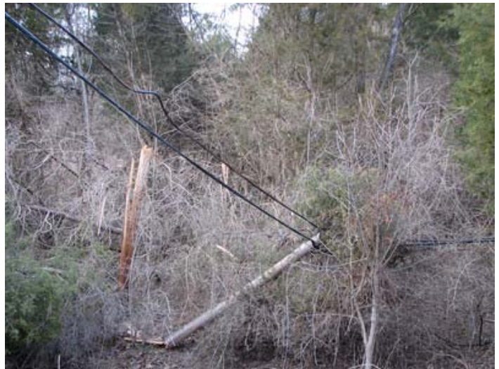
Snapped poles were across roads throughout Elk Lake. (Photo by Sam Altman)
